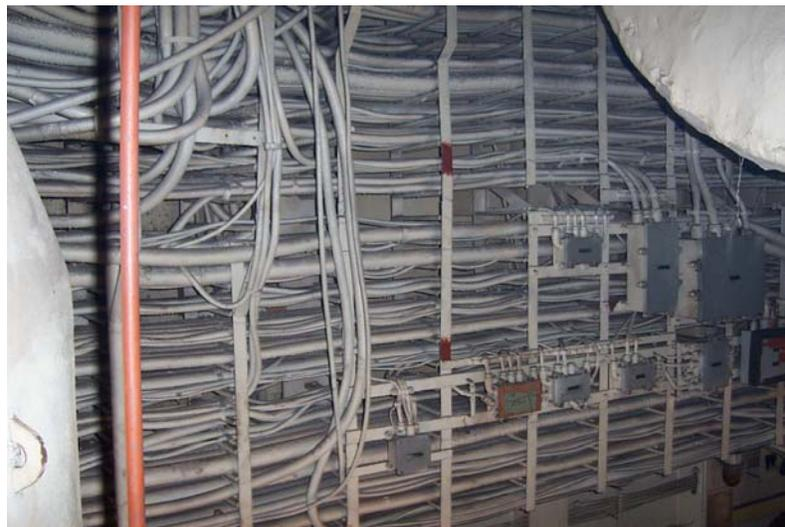
**Figure 3 Cable trays in auxiliary machine room.**
